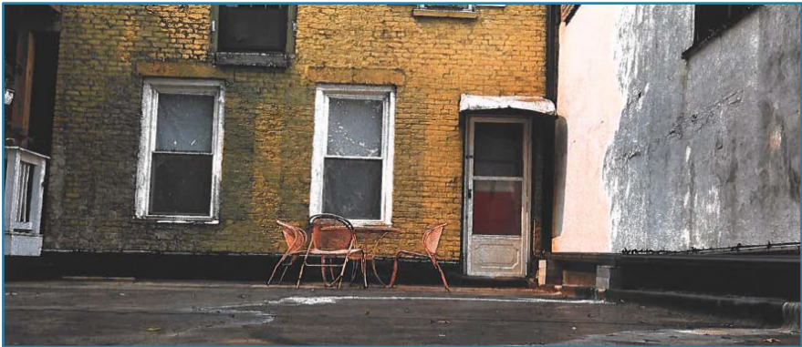
Above: Current back façade
