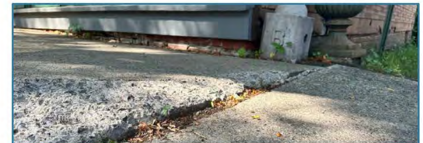
Above: Existing condition between Warren & Franklin Sts.
