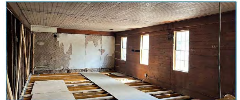
Above: Current condition, 2 nd floor
