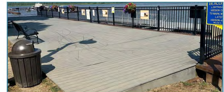
Above: Existing boardwalk condition
