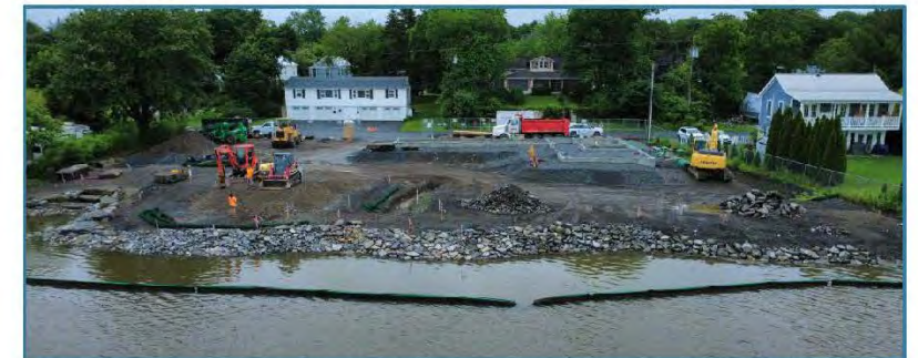
Above: Aerial of site condition
