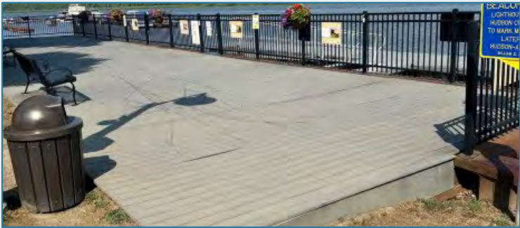
Above: Existing boardwalk condition
