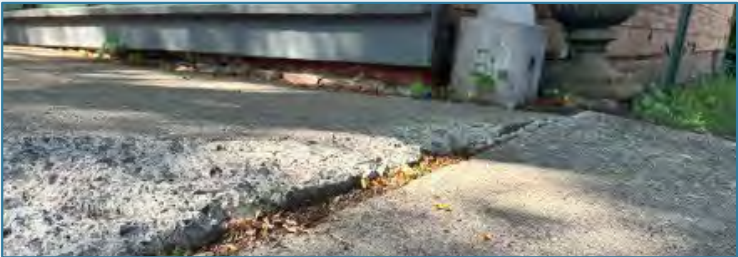
Above: Existing condition between Warren & Franklin Sts.
