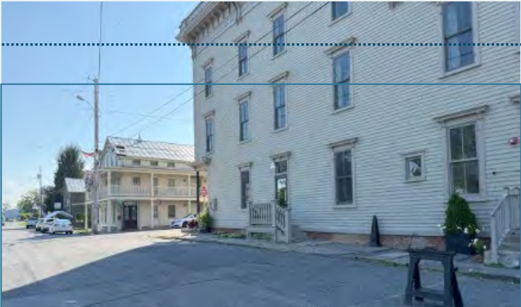
Stewart House exterior
