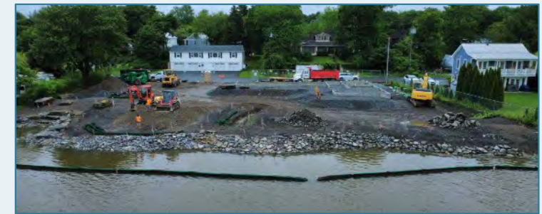
Above: Aerial of site condition
