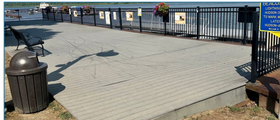
Above: Existing boardwalk condition
