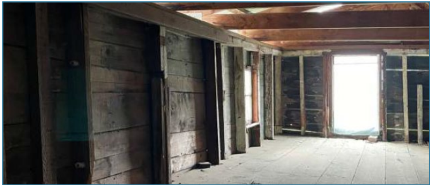
Above: Interior view of loft, current condition
