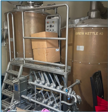
Above: Interior image of tanks
