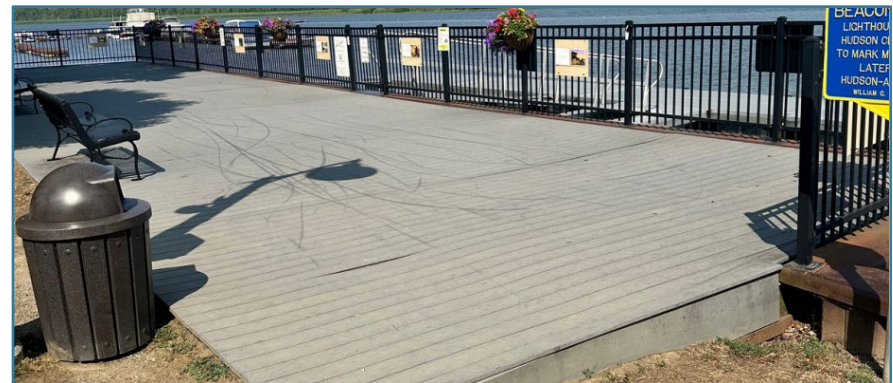
Above: Existing boardwalk condition
