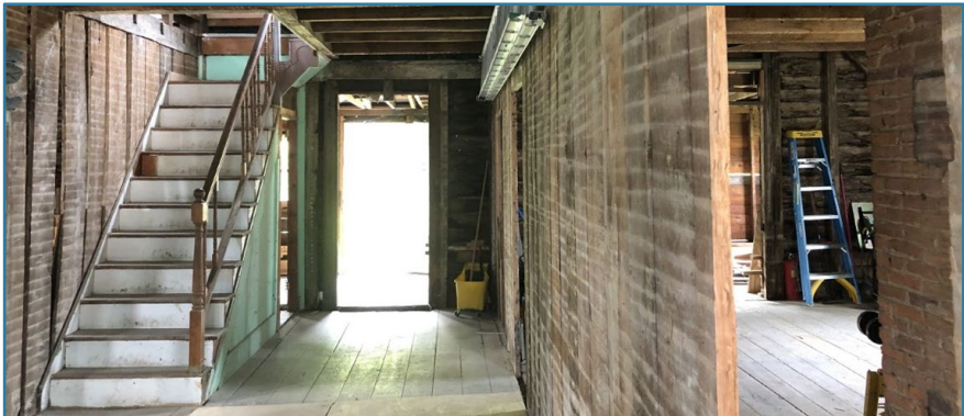
Above: Interior view, current condition
