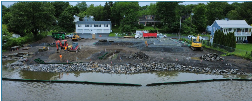
Above: Aerial of site condition
