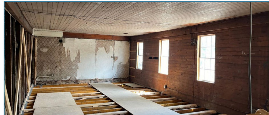
Above: Current condition, 2 nd floor
