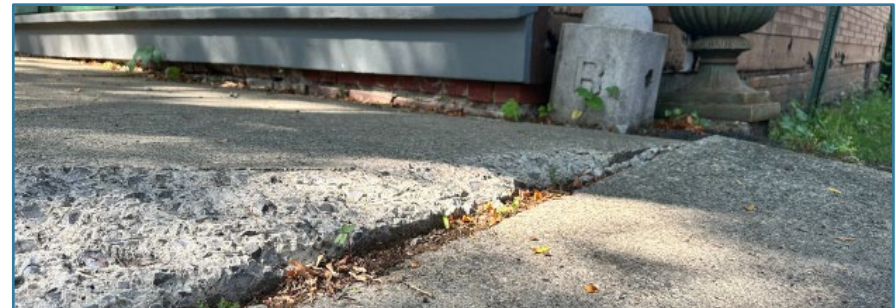
Above: Existing condition between Warren & Franklin Sts.
